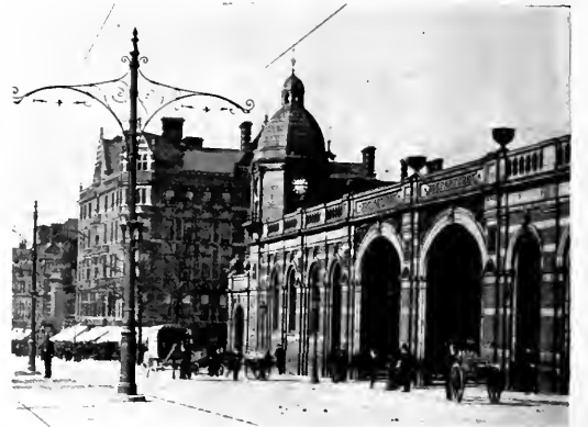
FIG. 2.—EXTERIOR OF POWER STATION.
